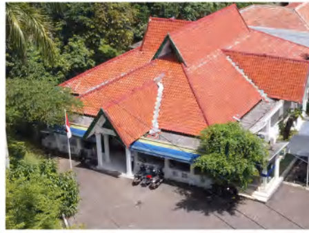
Kantor Jatiluhur Valley Resort Hotel Business Unit Office
