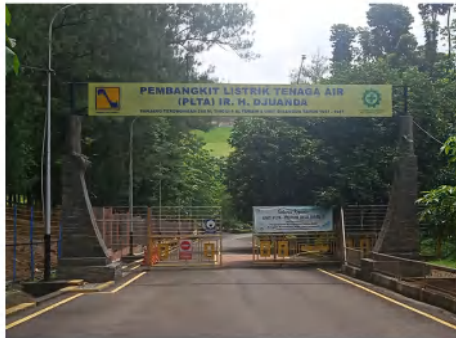
Kantor Unit PLTA Hydropower Unit Office
