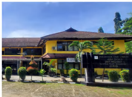
Kantor Unit Wilayah II Regional Unit Offices II
